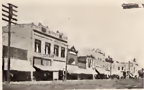
VILLARD STREET, Looking East, DICKINSON, N. D.
